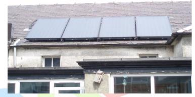
by a 500 litre tank and still meet the school's hot water demands. In addition, he took advantage of the fact that the school had a well protected south facing roof, facing into the eco garden, which could be utilised for solar thermal panels. He obtained 50% match funding for the project under the LCBP2 funding scheme, and the solar panels and associated visual display unit were installed in March 2009.
