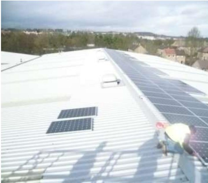
**Equipment:** 3 x Air to Air source heat pumps 10kW ceiling mounted with 30kWhp Suntech 250kWh PV panel installation.
