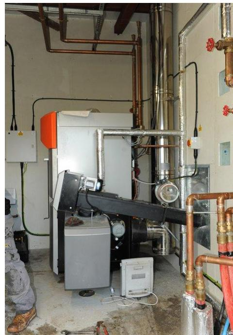
**Equipment:** 1 x 50kW Guntamatic power chip boiler, 1 x 100kW Guntamatic power chip boiler, 5000 litre accumulator tank, 2 x 48m<sup>3</sup> capacity fuel stores with 4m spring agitators and auger delivery.
